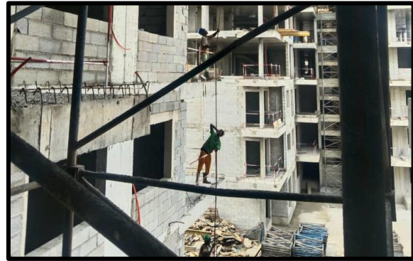
Figure 25 : Image illustrative du transport manuel du ferrailage passif
