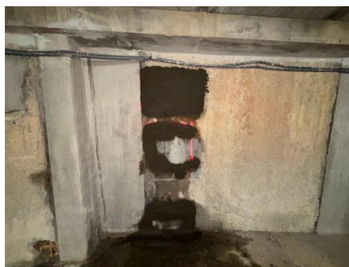
Figure 56 : Application maxrest panneau P3
