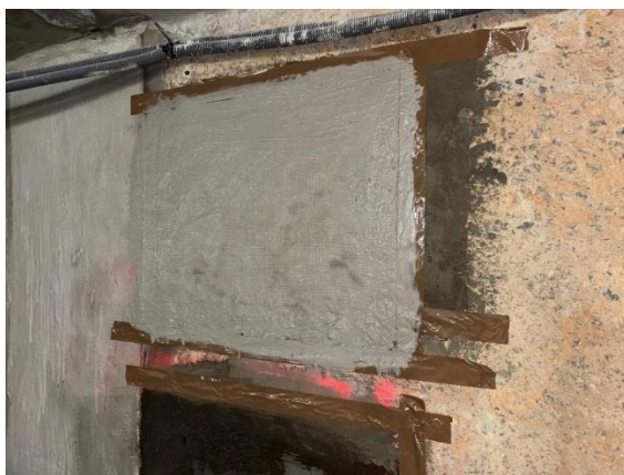
Figure 61 : Application couche finale Maxseal panneau P3
